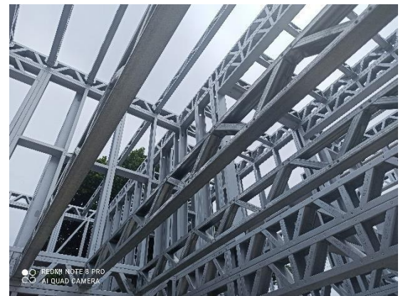
Figure 3: Floor joists in the building
