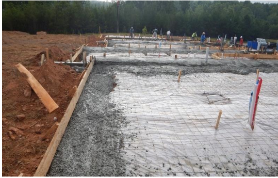
Figure 4: Slab on Grade (Kampert, 2021)
